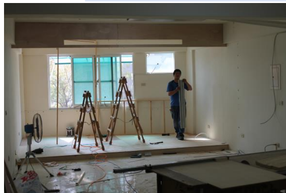
Remodeling work for new church auditorium.
